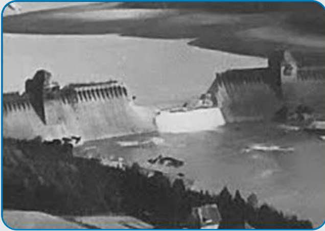
(Start of Banqiao Reservoir Dam breach)
