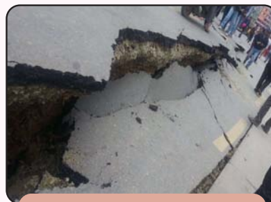
Six-lane highway, Bhaktapur
